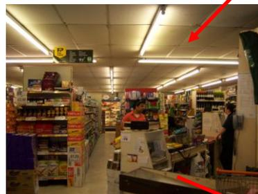
IP camera with 2-way audio is sited at the most vulnerable area(s) in the premises – in this case over the till adjacent to the tobacco and drinks sections (effective radius approximately 15m)
